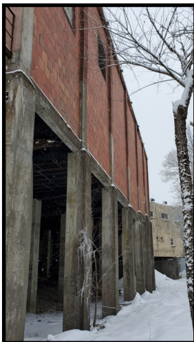
Looking from the NE corner of the building
